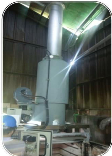
2 COMBUSTION CHAMBER INCINERATOR
